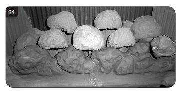
8.20 Place the left hand small coal in the recess between the flame baffle and the front coal, see Diagram 25.
