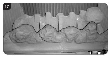
8.13 There are three sizes of coal used. Small x3, medium x4 and large x1. For identification, see Diagram 18.
