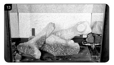
7.6 Place the foot of Log C into the rear left hand corner. The long flat edge rests against the side of the firebox and the log touches the back panel. The top of the log rests on Log E, see Diagram 14.
