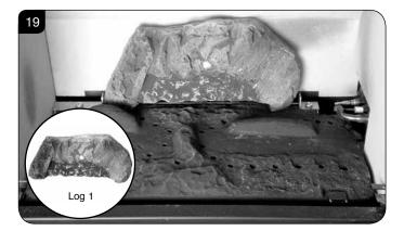
7.12 Place the second log into the left hand groove on the burner tray, see Diagram 20.The log should butt up against the raised molding and the left hand side liner.
