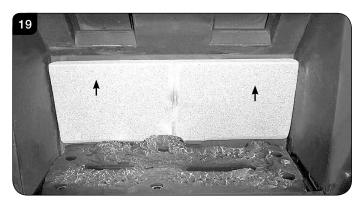
4.28 With the liners and baffle removed the firebox is clear for cleaning and maintenance, see Diagram 20.
